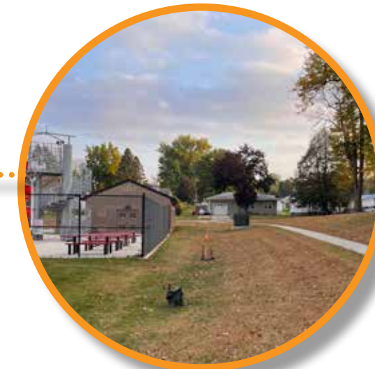
Swale on the west side of the pool is capturing water from the hillside and pool area
