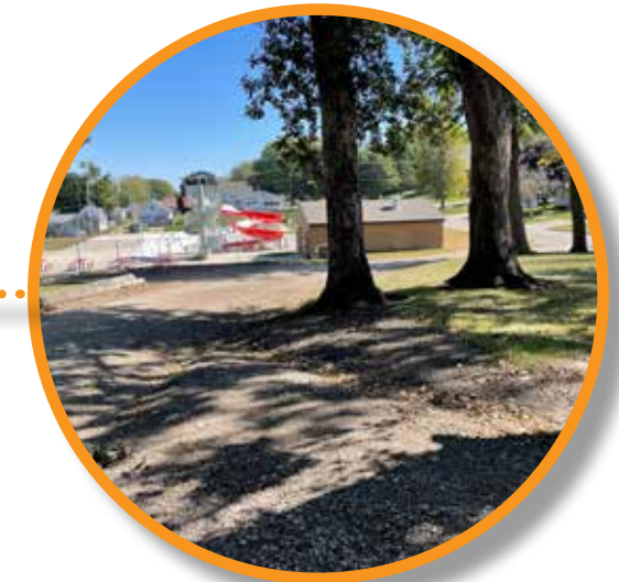
Ruts have developed in the gravel drive due to stormwater erosion
